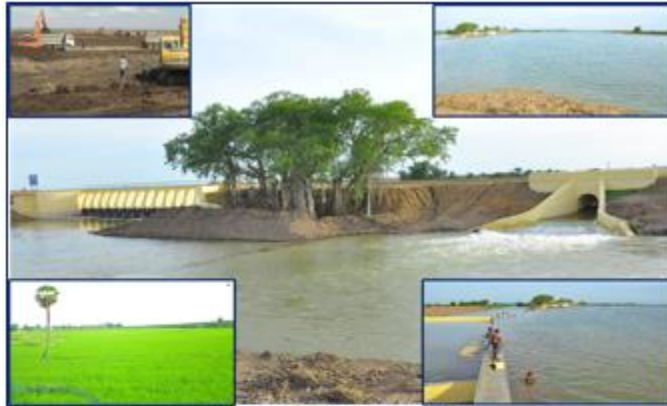
WALAJAH LAKE DE-SILTING AND ALLIED WORKS
