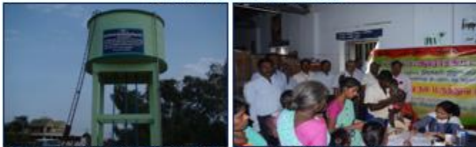
80,000 LITRE OVERHEAD WATER TANK - VALARUTHU
